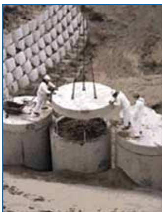
Waste materials with low levels of radiation are stored in secure containers. Then they are buried in a landfill.
