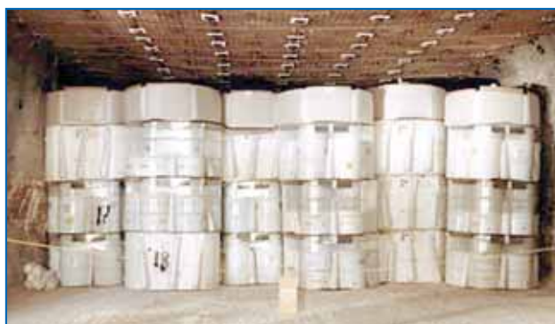
Radioactive products from nuclear power plants are very hazardous. The Waste Isolation Pilot Plant (WIPP) is a site in New Mexico where the United States government is developing safe storage for harmful radioactive wastes. Large rooms 2150 feet (almost one-half mile) underground house the waste in secure barrels.
